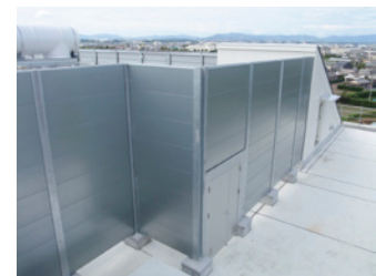
The soundproof wall
