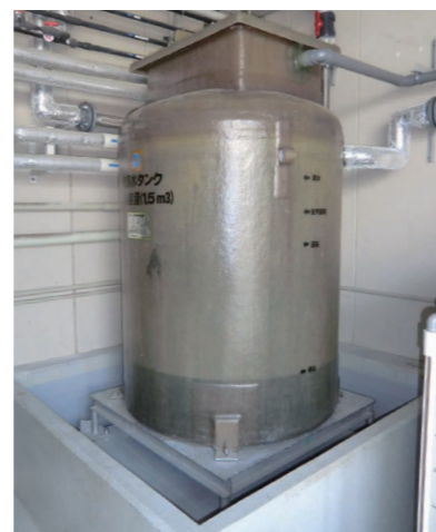
Tank relocated aboveground
