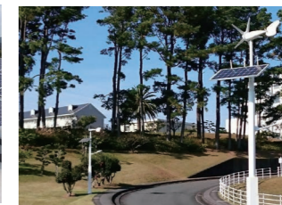
Wind and solar hybrid outdoor lights (Central Research Laboratory)
