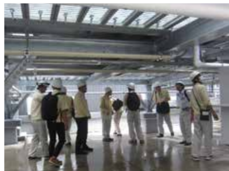
Underfloor inspection of waste gas treatment equipment
