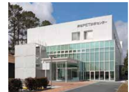
Hamamatsu PET Diagnostic Center
